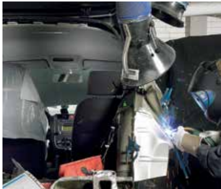
MIG/MAG welding in sheet metal
